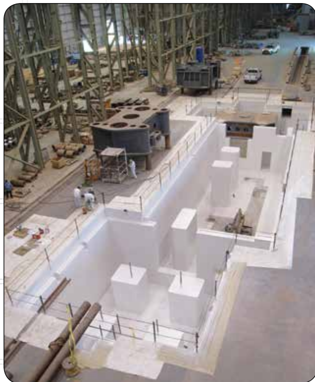
Foundation for the new forge press
